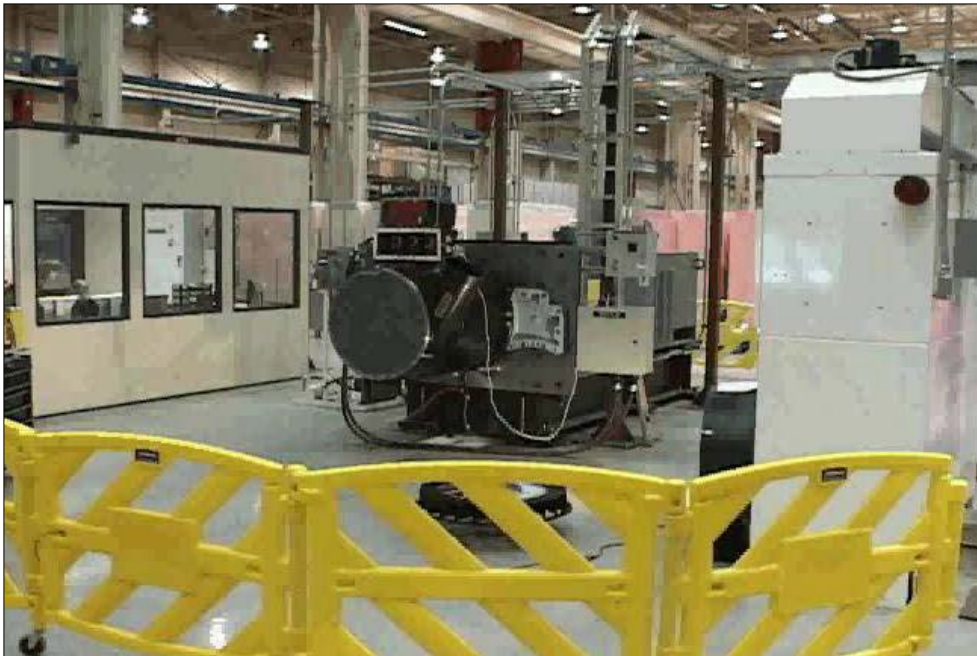
Figure 18. Dynamometer used for generator tests at Clipper Turbine Works plant in Cedar Rapids, Iowa.
