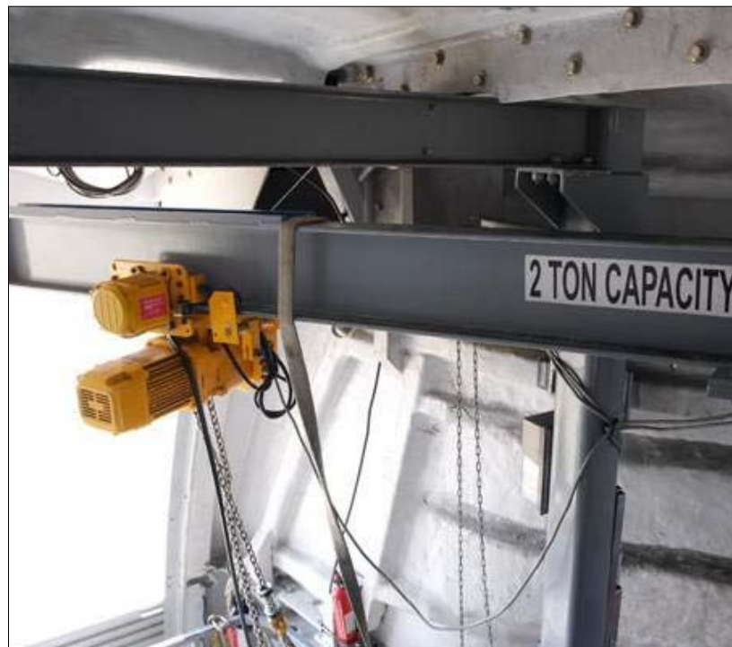
Figure 7. The 2-ton jib crane in the C93 Liberty turbine
