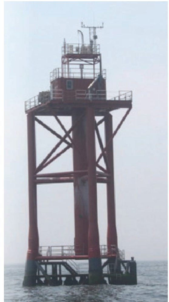
Meteorologic equipment on Ambrose light station collects the wind and wave data used for the reference database.
