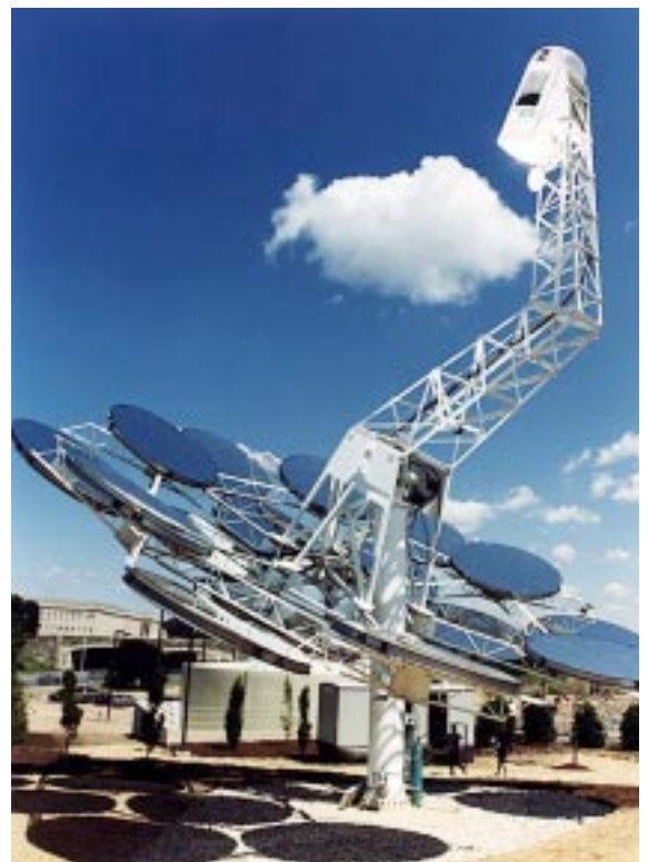
Figure 1. Dedication of the dish/Stirling system at the Pentagon in Washington, D.C. Shown in the picture are the concentrator and the STM 4-120 Stirling engine/generator package.
