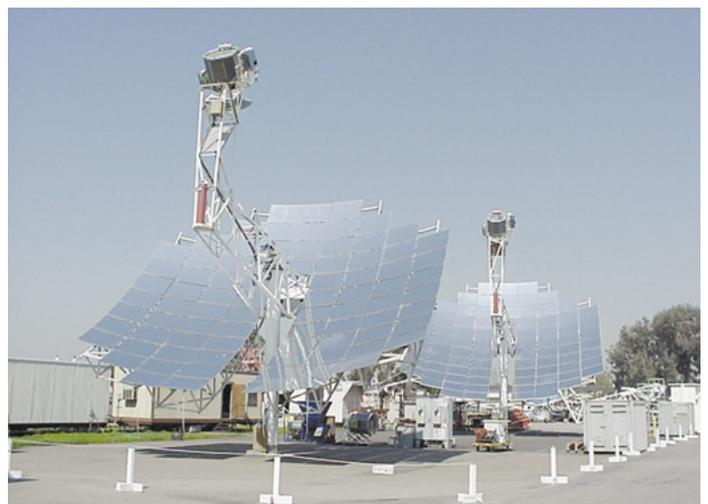
*Solar dish systems are the most efficient solar systems in the world. They provide economical power for utility line support, distributed, and remote applications, and are capable of fully autonomous operation. Sized between 10 and 25 kW per dish, systems can be deployed individually for water pumping or village power applications or grouped to form megawatt-scale power plants.*
