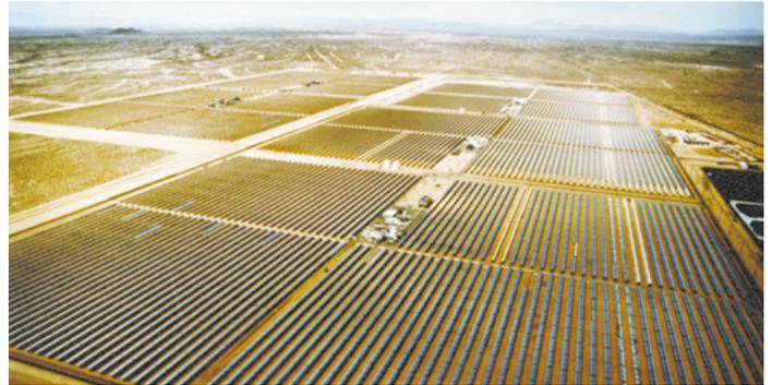
*354 MW of SEGS plants continue to operate successfully on the California power grid. Annual output of the plants has increased by 35% as plant operations have improved during the past 10 years, and operation and maintenance costs have correspondingly dropped 40%. These plants have demonstrated the ability of CSP to meet utility requirements. Several domestic and international projects are currently being planned.*
