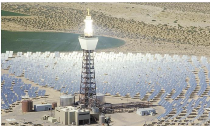
*Solar Two successfully demonstrated the power tower concept, including the capability to store energy economically for dispatch at periods of peak demand. U.S. industry is building the first commercial power tower using this technology in Spain and simultaneously investigating near-term opportunities in the United States.*
