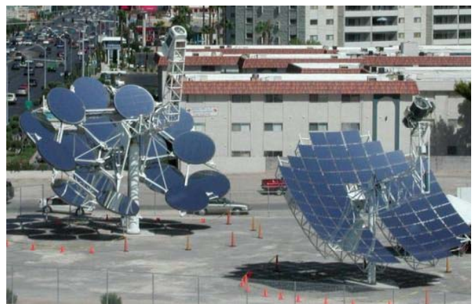
Figure 4. 25 kW Dish/Engine Systems
